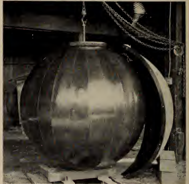
Spherical molds for concrete storage tank for flammable liquid fuels. Cement is poured between the molds and allowed to stand for 12 hours.
